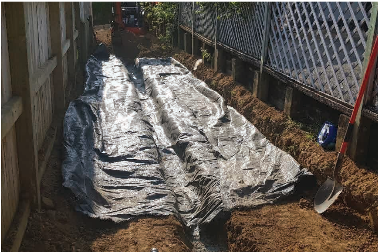
Figure 11. Service trench with geotechnical cloth covering R11/3251 for protection.
