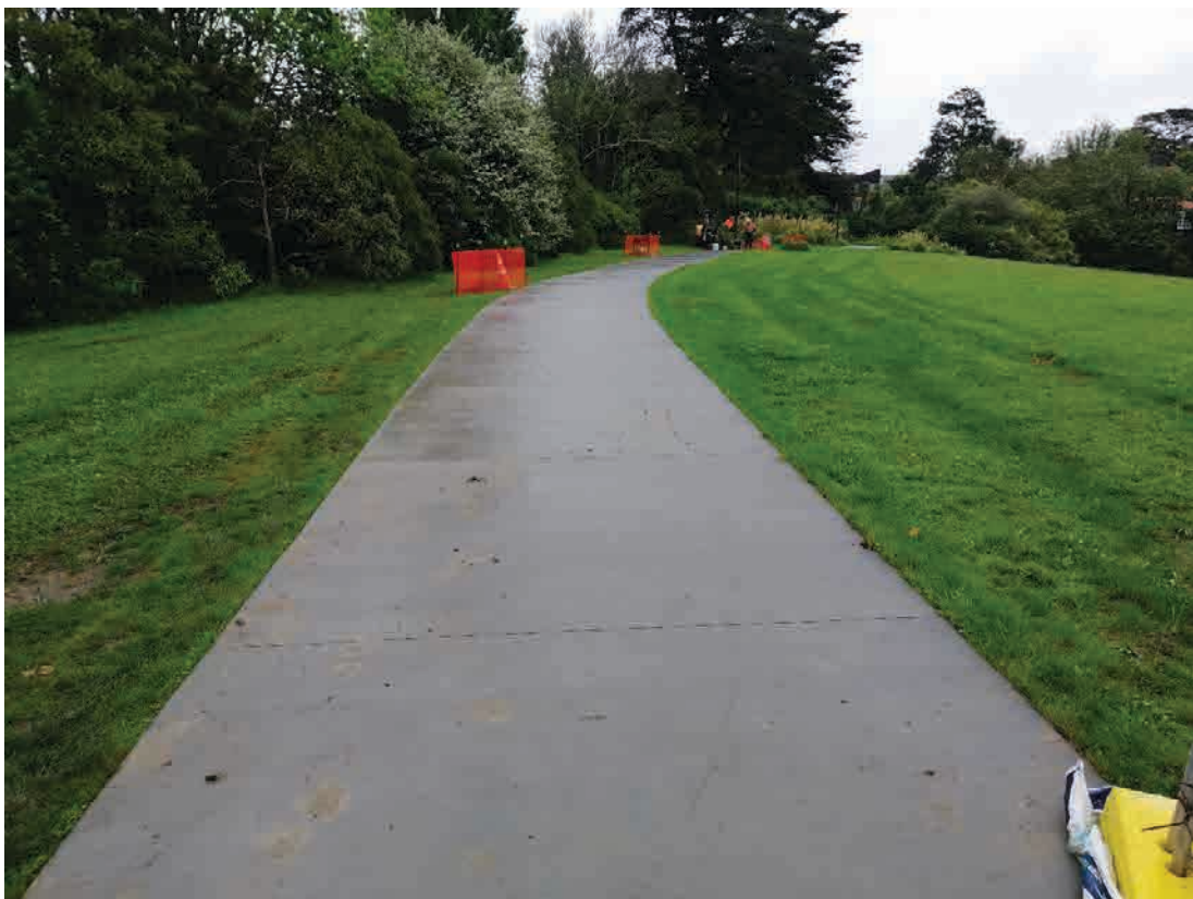
Figure A3. View of the new feeder path facing south.
